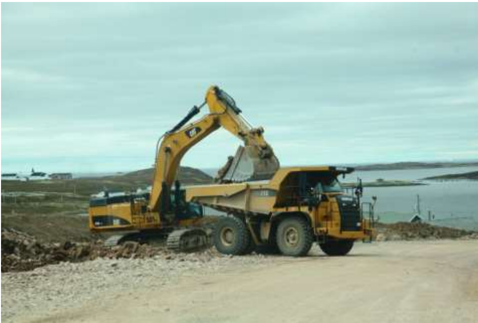
Moving rocks from trench to roadbed
