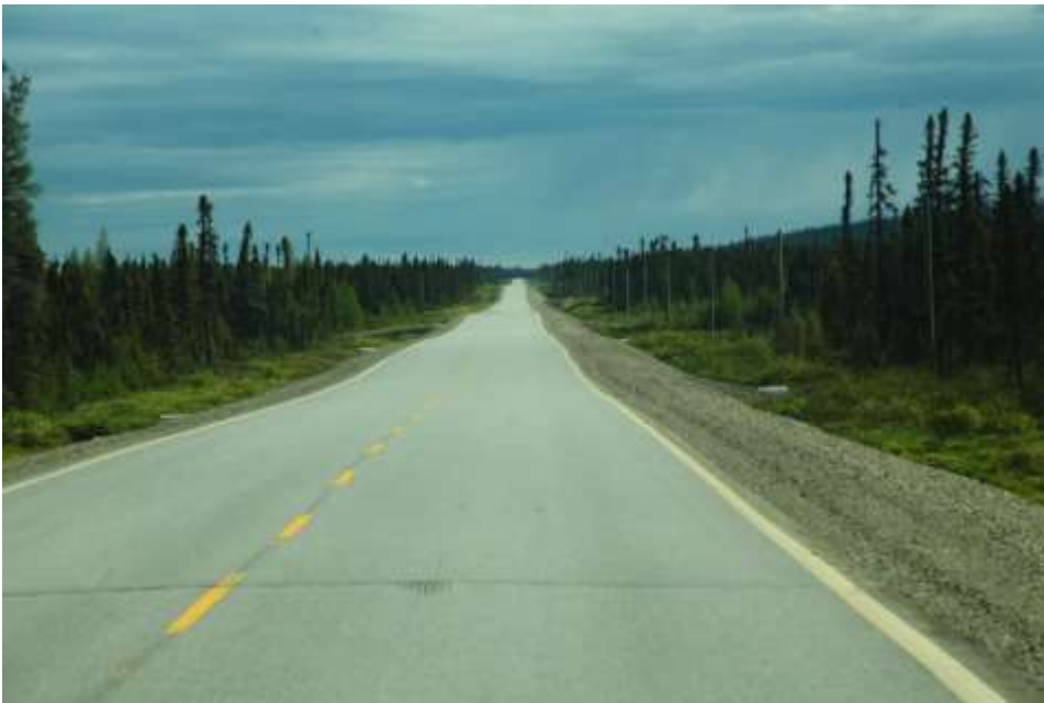
Excellent paved section of Trans-Labrador Highway
