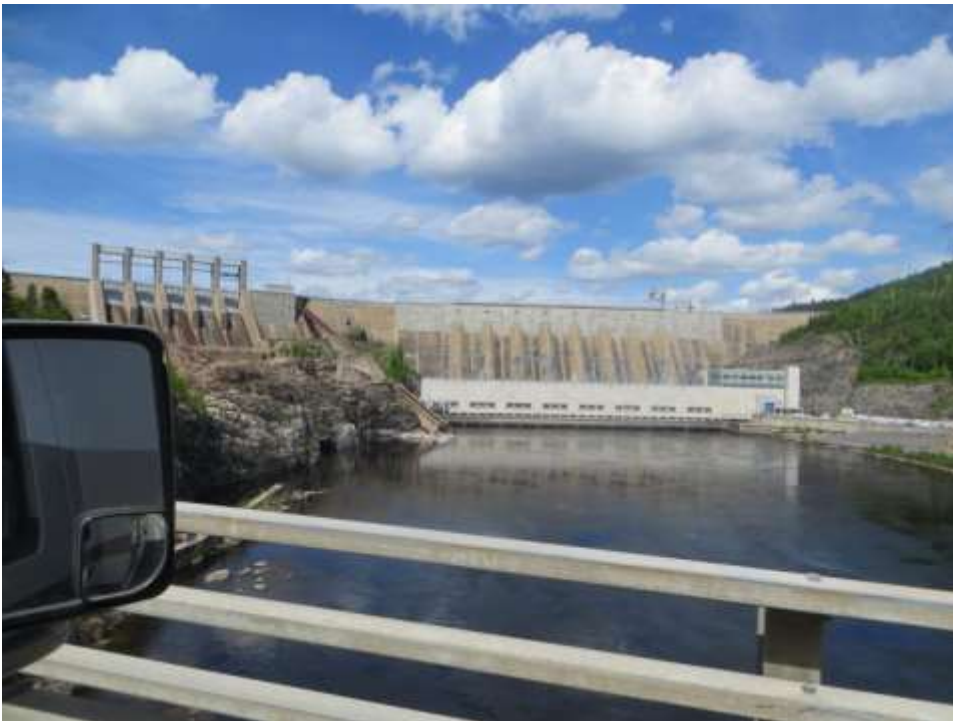
Manic-5 Dam from the bridge over Manicouagan River
