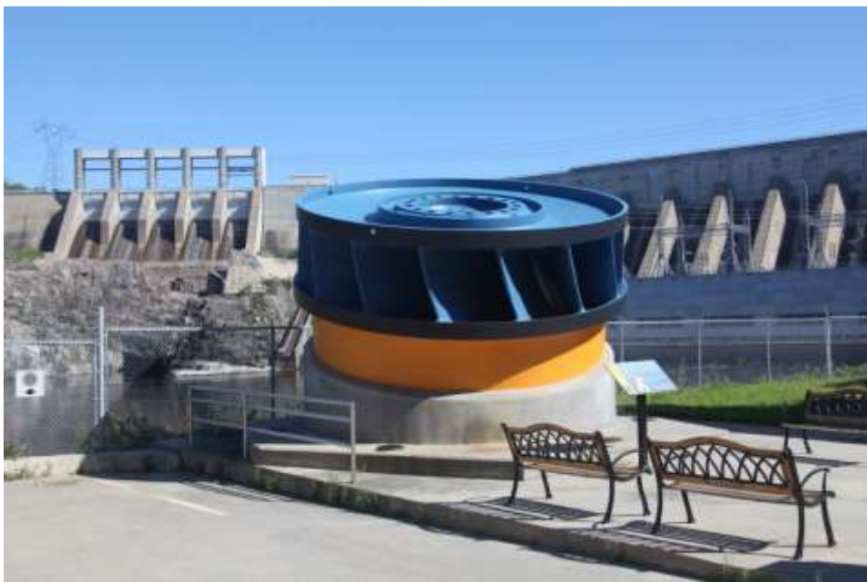
Manic-2 in the background; unused turbine in foreground
