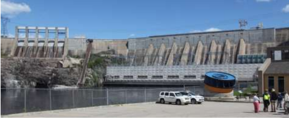
Spillway and Manic-2 dam
