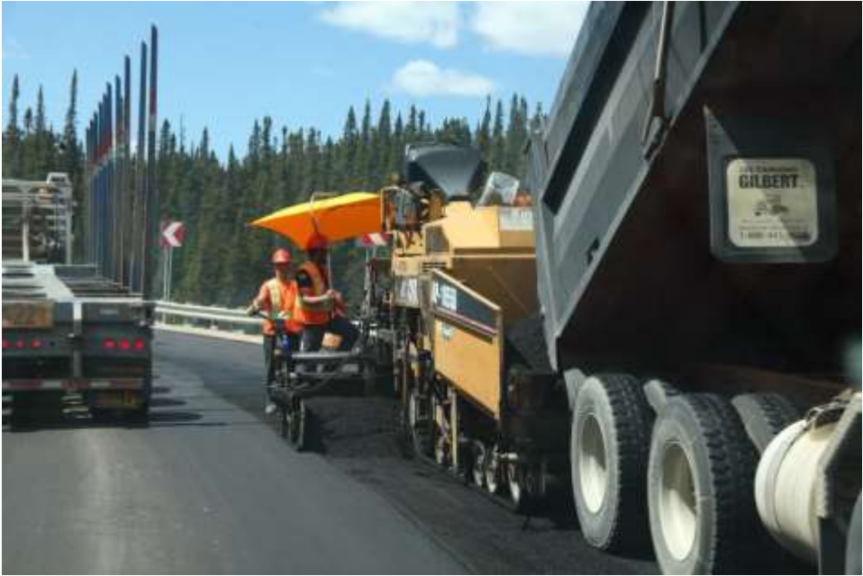
Repaving the highway
