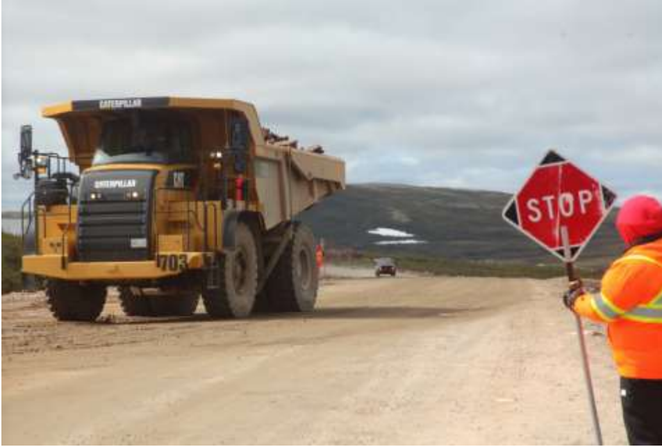
Road rebuilding on Trans-Labrador Highway
