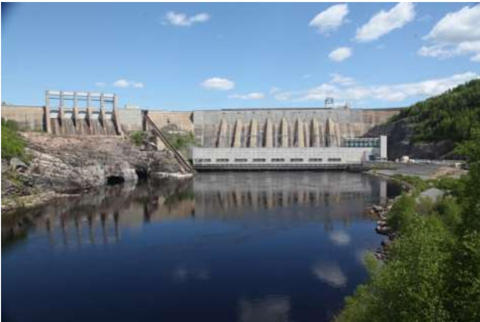
Spillway and Manic-2 dam
