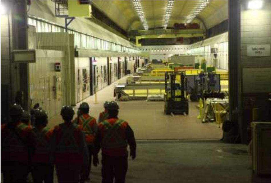
Entering the control room
