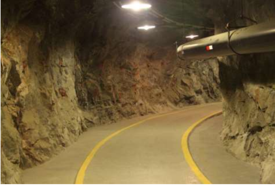
Granite tunnel from elevator to transformer room
