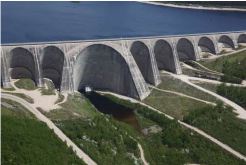
Manic-5 showing large central buttress
