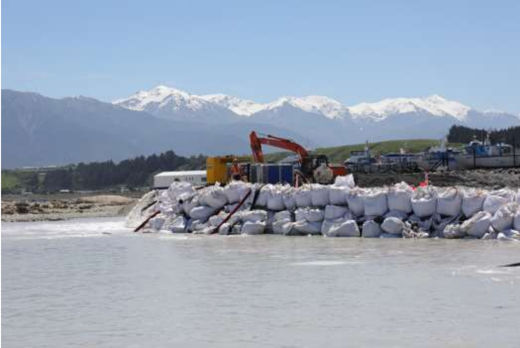
Construction of new dock at Kaikoura since the earthquake
