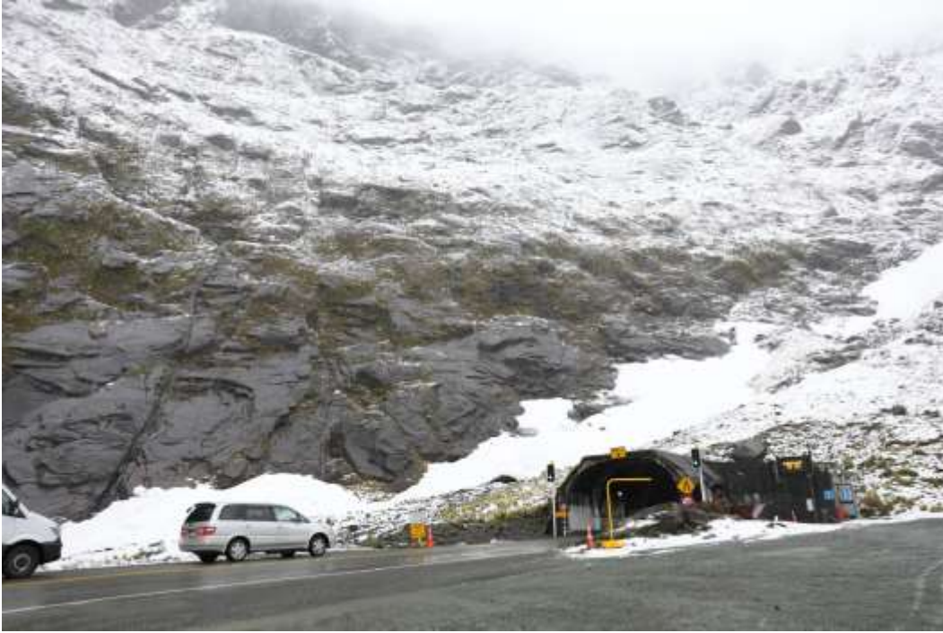
Homer Tunnel, elevation 3030 ft. descending to 2630 ft.
