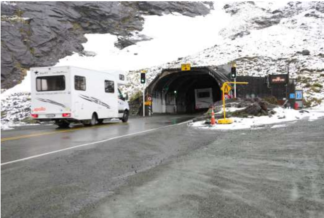
A traffic light controls passageway through one-way Homer Tunnel
