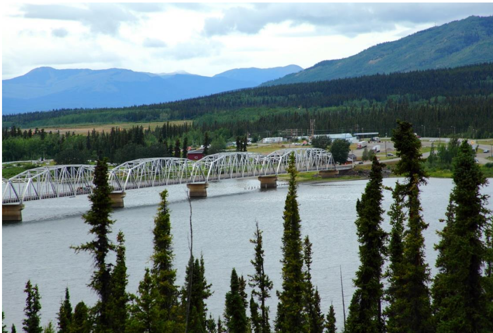
1917-ft. Nisutlin Bay bridge, the largest span on the Alaska Highway
