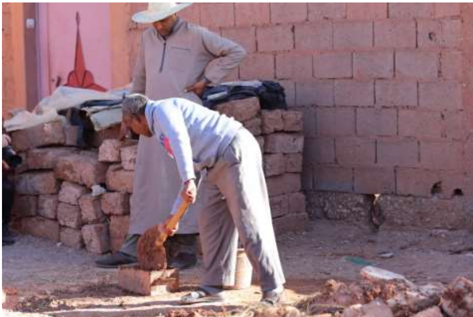
Shoveling adobe into mold
