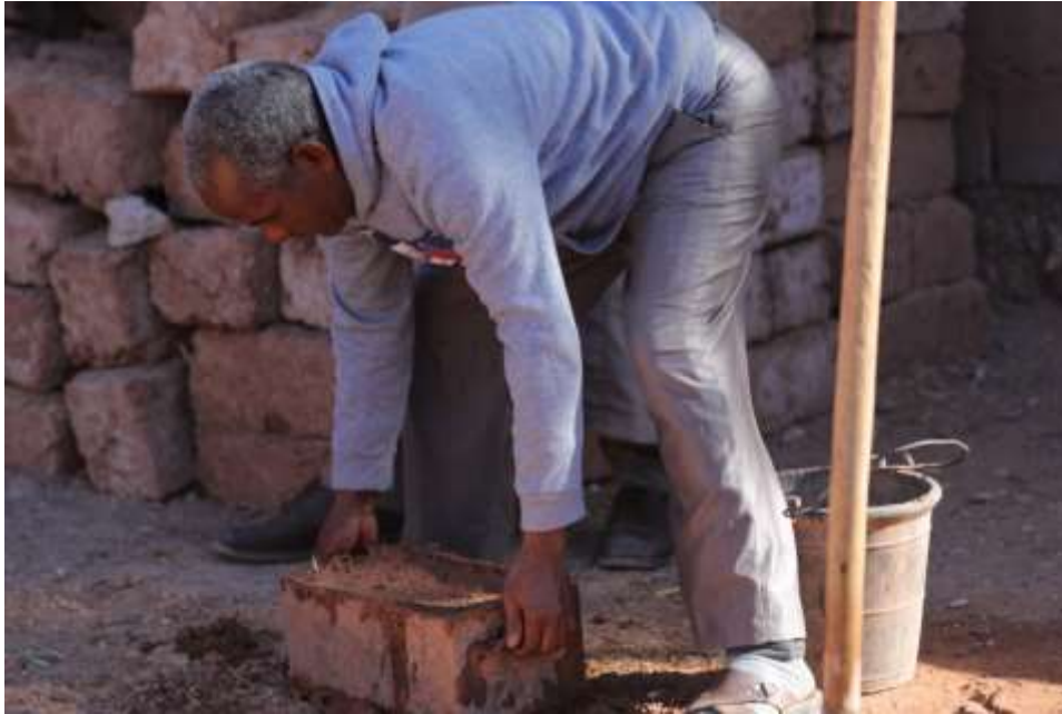
A new brick
