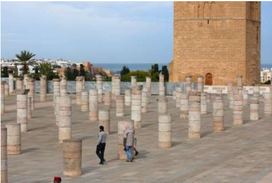
Some of the 348 original columns
