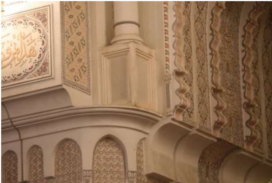
Loud speakers are hidden within the wood paneling in the upright rectangular box
