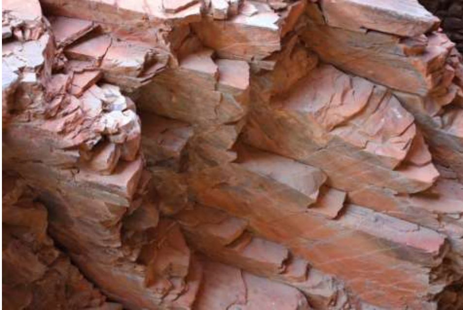
Looking up at the sharply defined breaks from which rock fell
